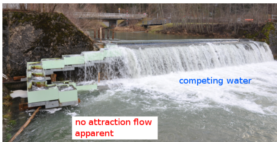
Figure 35: Steffstep on 12.01.16 with a high discharge of 10 m 3 /s
