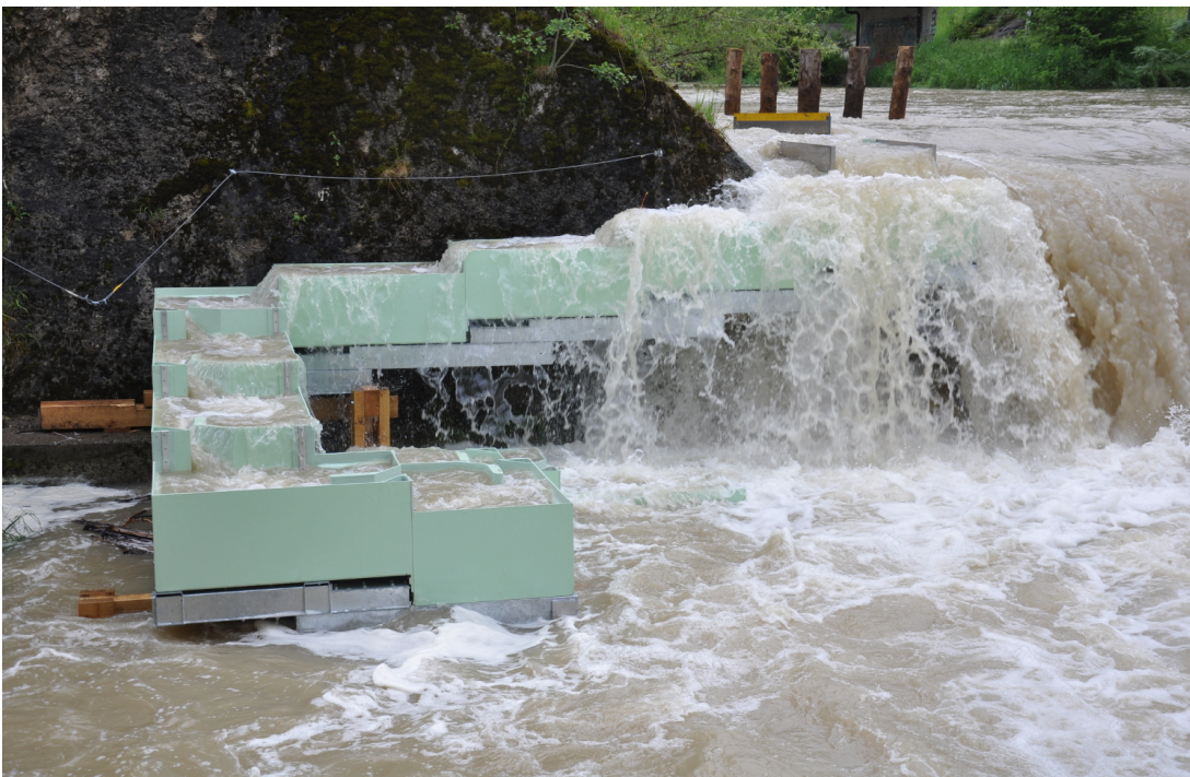
Figure 11: Flood on 26.05.15 with 32 \text{ m}^3/\text{s}^* , the first and last pools are under water
